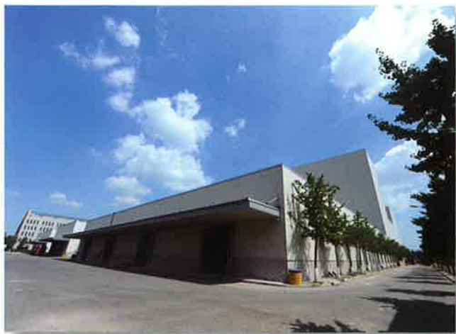
Figure 1: Outside view of the new plant
