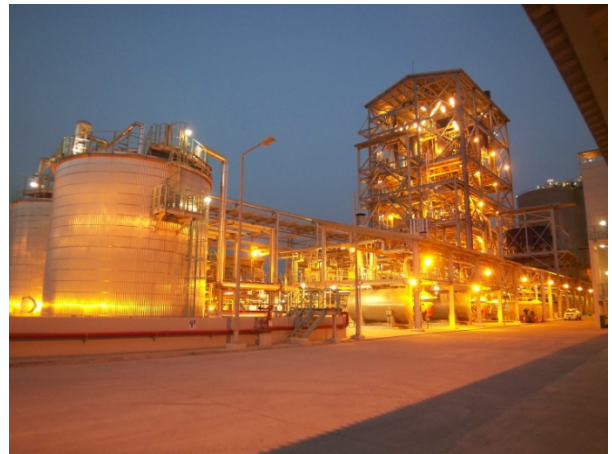
Fig 7: 60 t/h paste plant at Qatar Aluminium/Qatar
