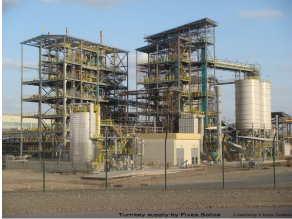
Fig 6: 36 t/h paste plant at Sohar Aluminium/Oman
