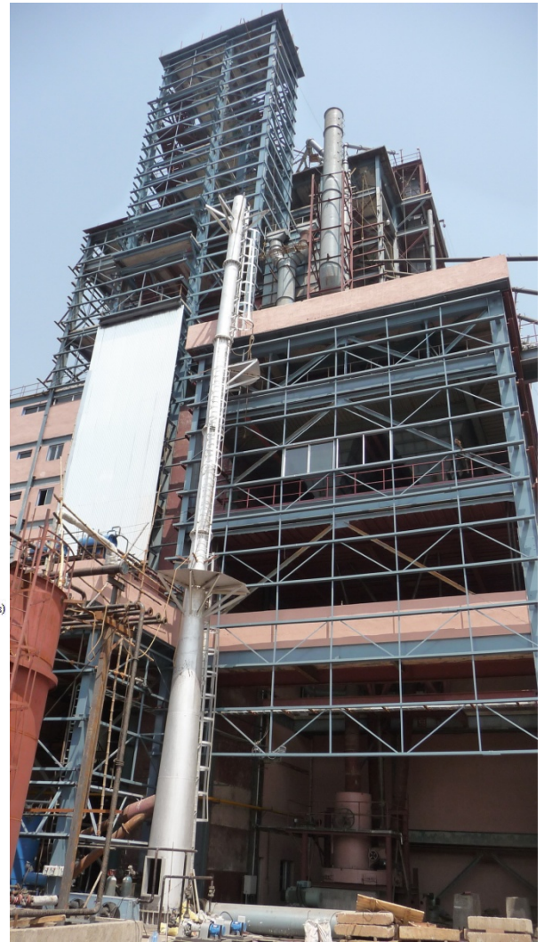
Fig 11: Paste plant at Graphite India Durgapur 2012
